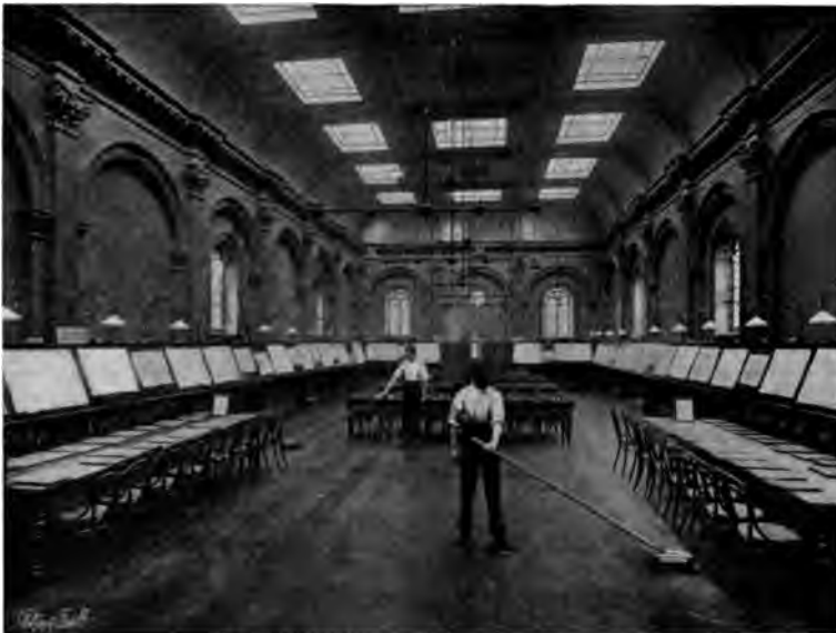
Fulham Public Library Reading Room. Floor Polished by Ronuk, Ltd.
